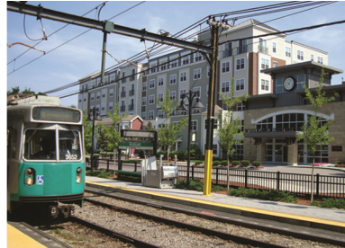
Arbor Point at Woodland Station, Newton, MA
