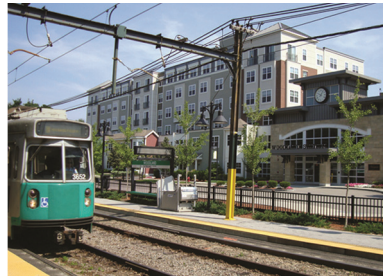
Arbor Point at Woodland Station, Newton, MA
